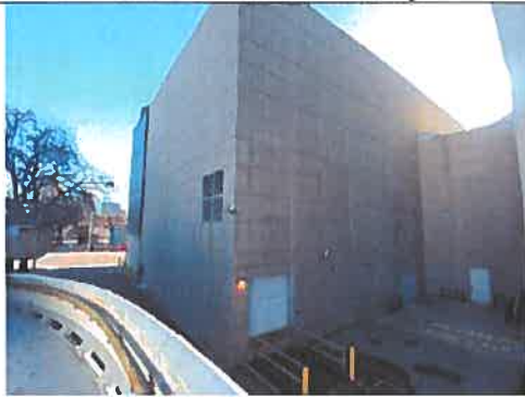
Southeast at Dock Area of DW Building
