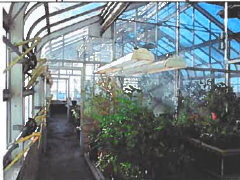
Greenhouse on Rooftop of MPM
