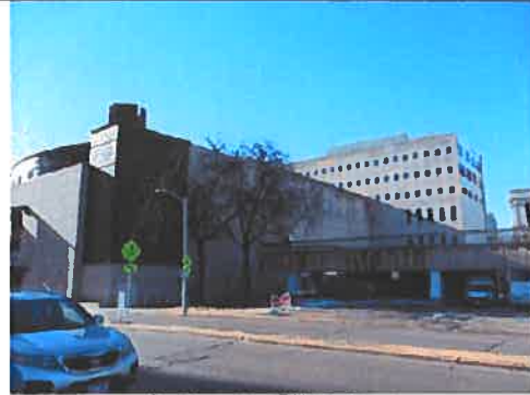
Southwest at DW Building
